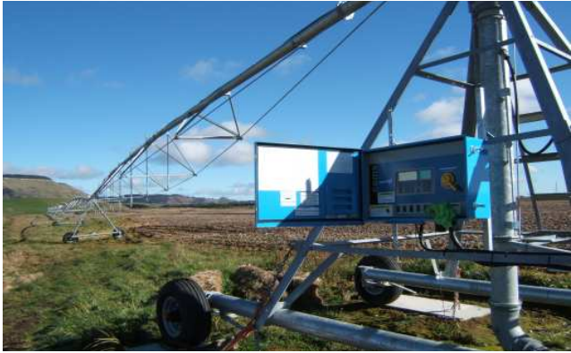
Fig. 5 One of many new centre pivot installations in NZ
